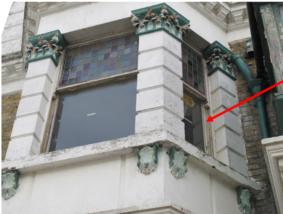
Figure 6 First Floor External Windows - Windows and window frames repeatedly grained in imitation of hardwood
