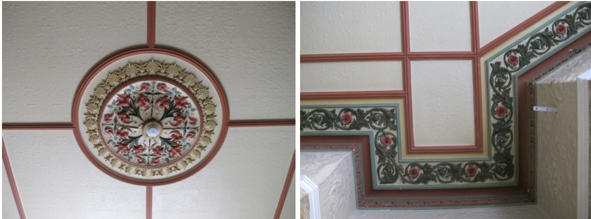
Figure 5 Reception Room (R0.01) Detail of decorative plaster mouldings on ceiling and cornice
