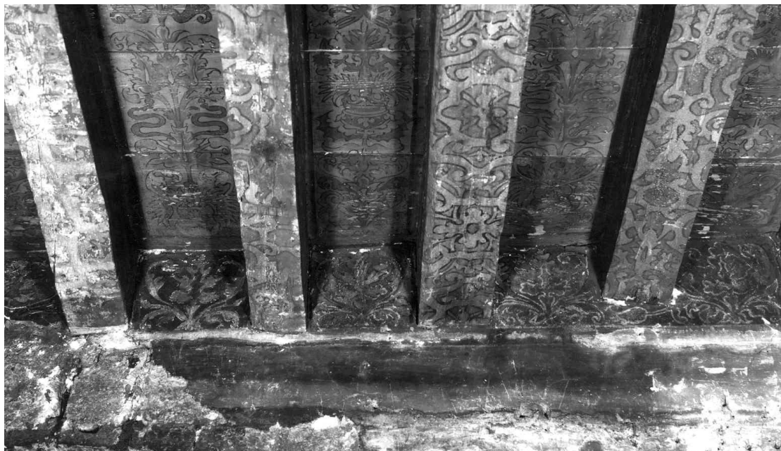
Figure 9 King James' Room - Ceiling, plaster frieze and wallface revealed
