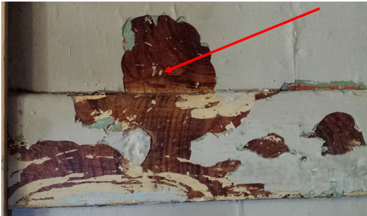
Figure 33 Orwell Room - Detail of graining exposed on salvaged elements in cupboard
