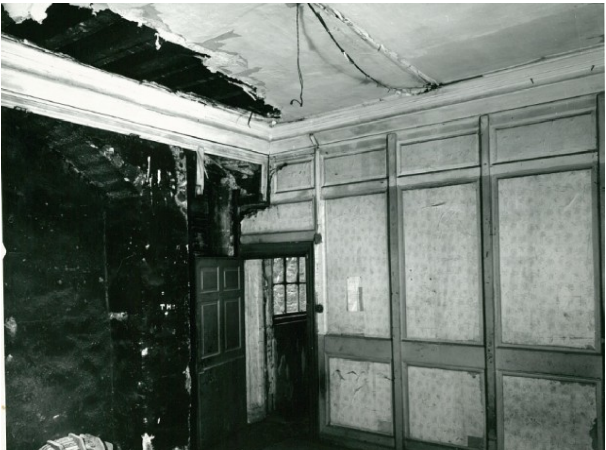
Figure 7 King James' Ceiling - North East Corner - 1960s
