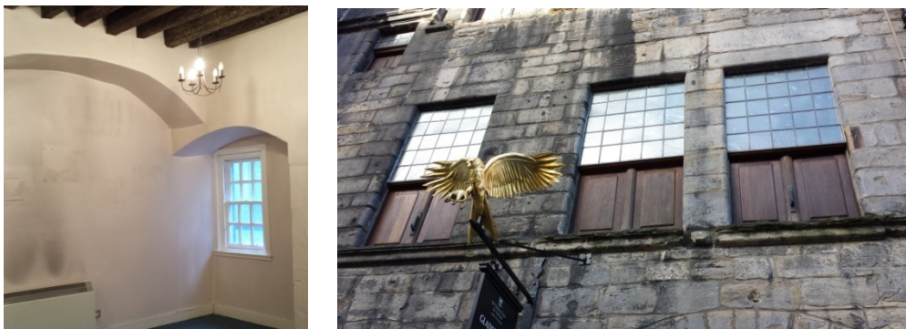
Figure 1 King James' Room SW Corner - SW Corner Sash Window - Examples of 16th Window
