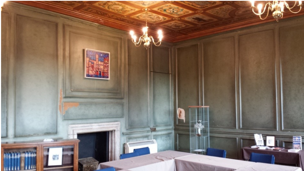
Figure 20 Geddes Room - Panelling thought to date from the late 17th century
