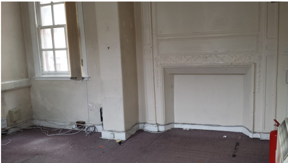
Figure 52 Ante-Room to Norie Room (F03) - South & North Walls
