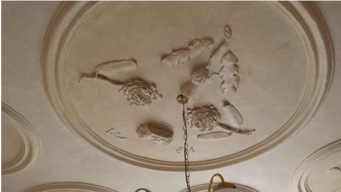
Figure 27 Norie Room - 17th Century Ceiling - Central Compartment
