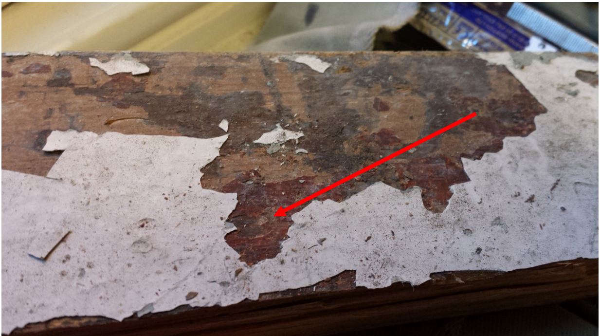
Figure 59 Room S0.8 Detail of surface of detach shelving - Traces of early graining (1 vibrant red) visible
