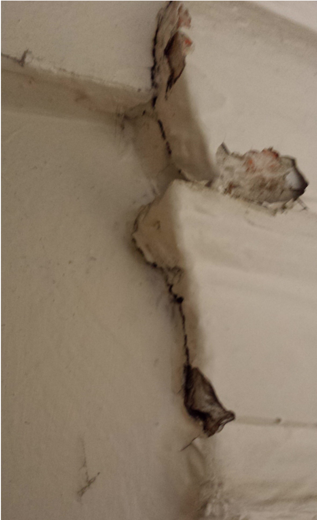
Figure 54 Room SO2 - Cornice and upper panel - paint build-up
