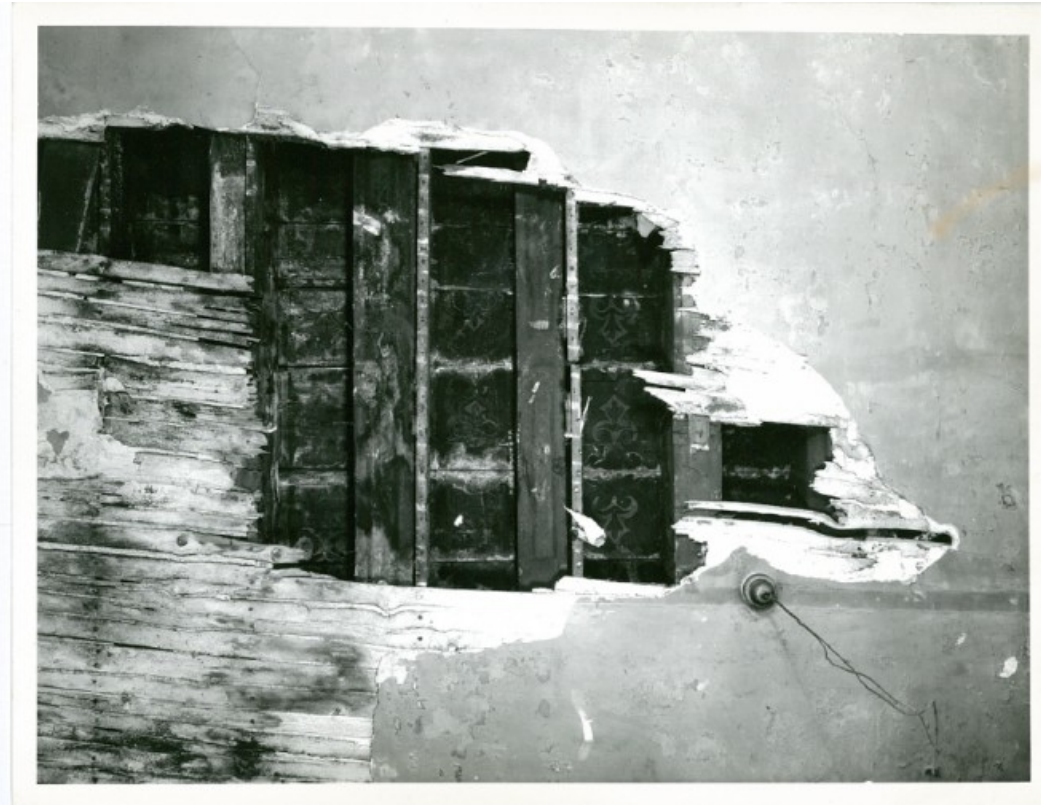
Figure 8 King James Room - Discovery of the painted ceiling
