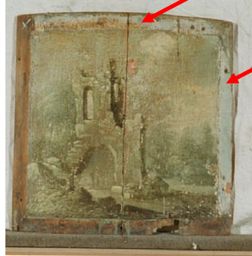
Figure 45 Norie Panels removed for conservation - Note exposed Light Blue at edges of the Norie landscapes which would have been exposed
