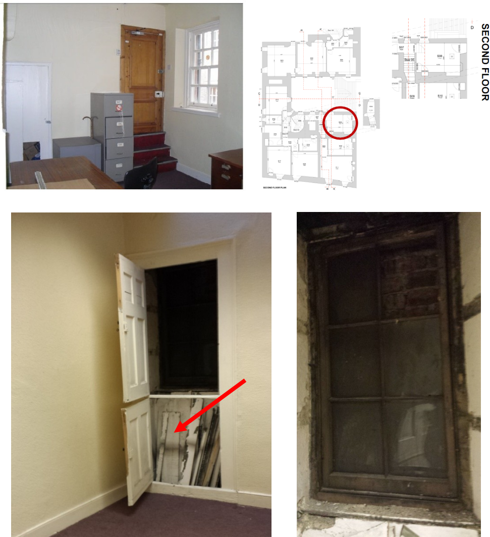
Figure 55 Room S0.8 - Window converted into a cupboard - East Wall NB Detatched17th painted boards
