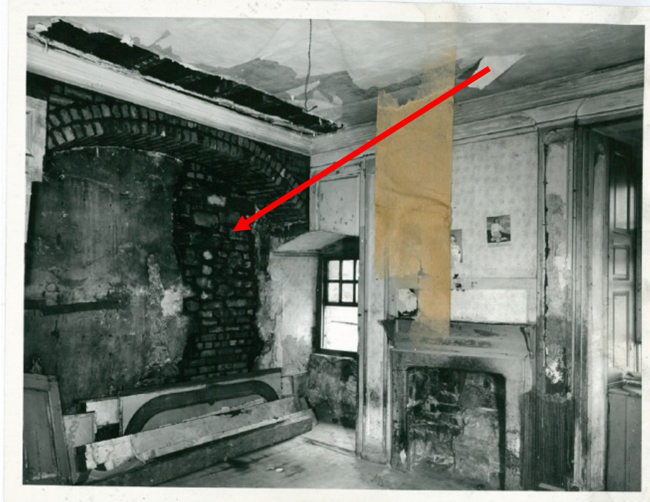
Figure 12 King James' Room - SW Corner - Evidence of blocked doorway
