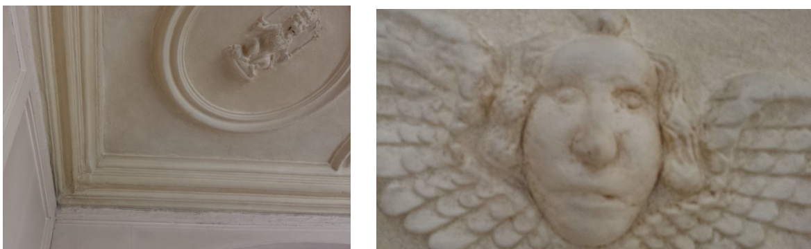
Figure 26 Norie Room - 17th Century Ceiling - Details
