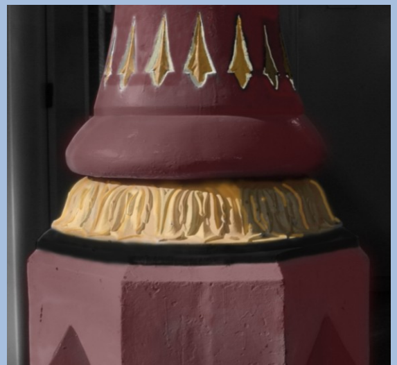
Figure 33 Gold paint (with glazes) applied to lower moulding and recesses
