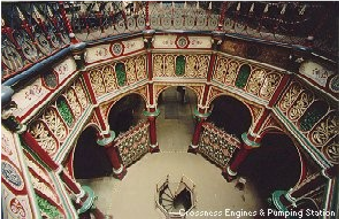
Figure 3 Crossness Pumping Station c.1980
