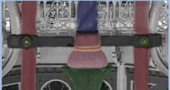
Figure 36 Structural supports- 1st Floor balustrade
