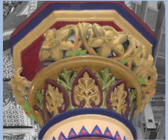
Figure 31 Gold paint (with glazes) applied to foliate mouldings
