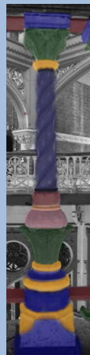
Figure 20 Dark blue on column of 1st Floor balustrade
