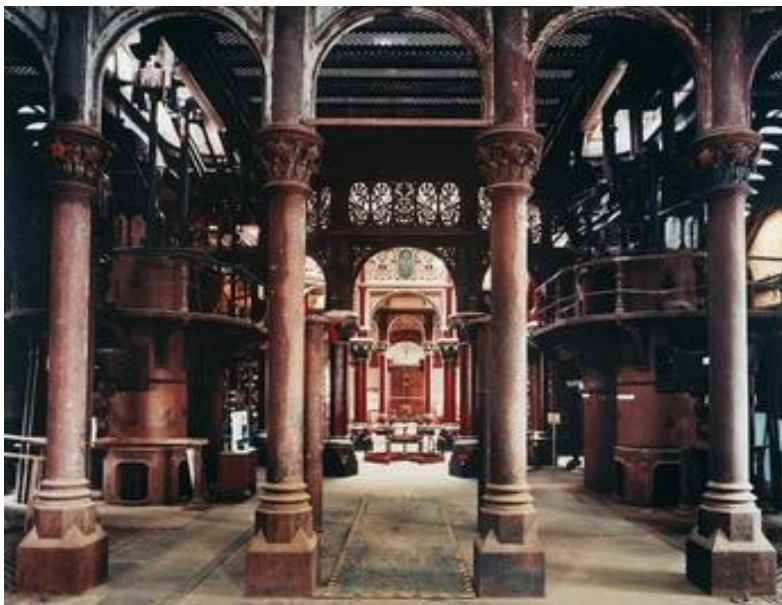
Figure 7 Crossness Pumping Station - General view of un-restored areas
