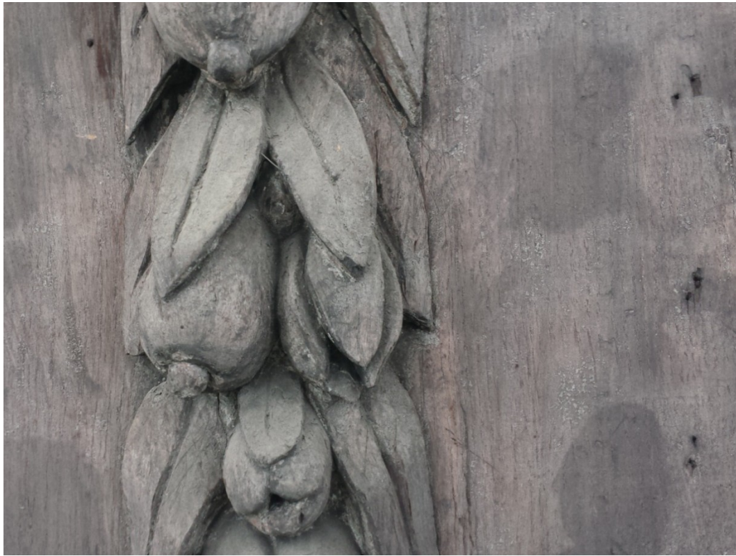
Figure 32 Interior of Cupola - Original joinery - stripped but traces of original paint are retained in mouldings
