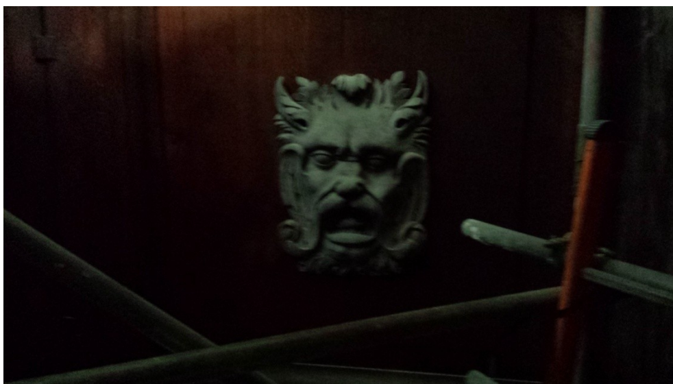
Figure 30 Interior of Cupola - Lower tier Grotesque Masks on replacement panelling.
