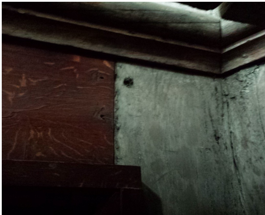
Figure 33 Interior Cupola – Junction of stripped original and replacement joinery - not painted
