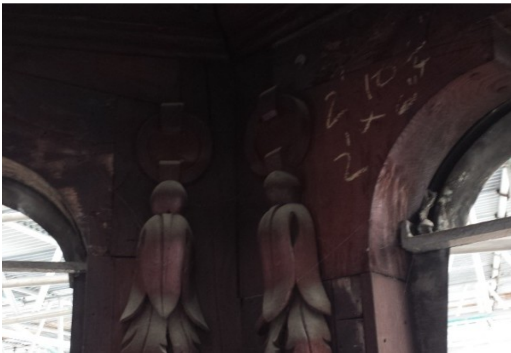
Figure 31 Sections of replacement joinery – western side
