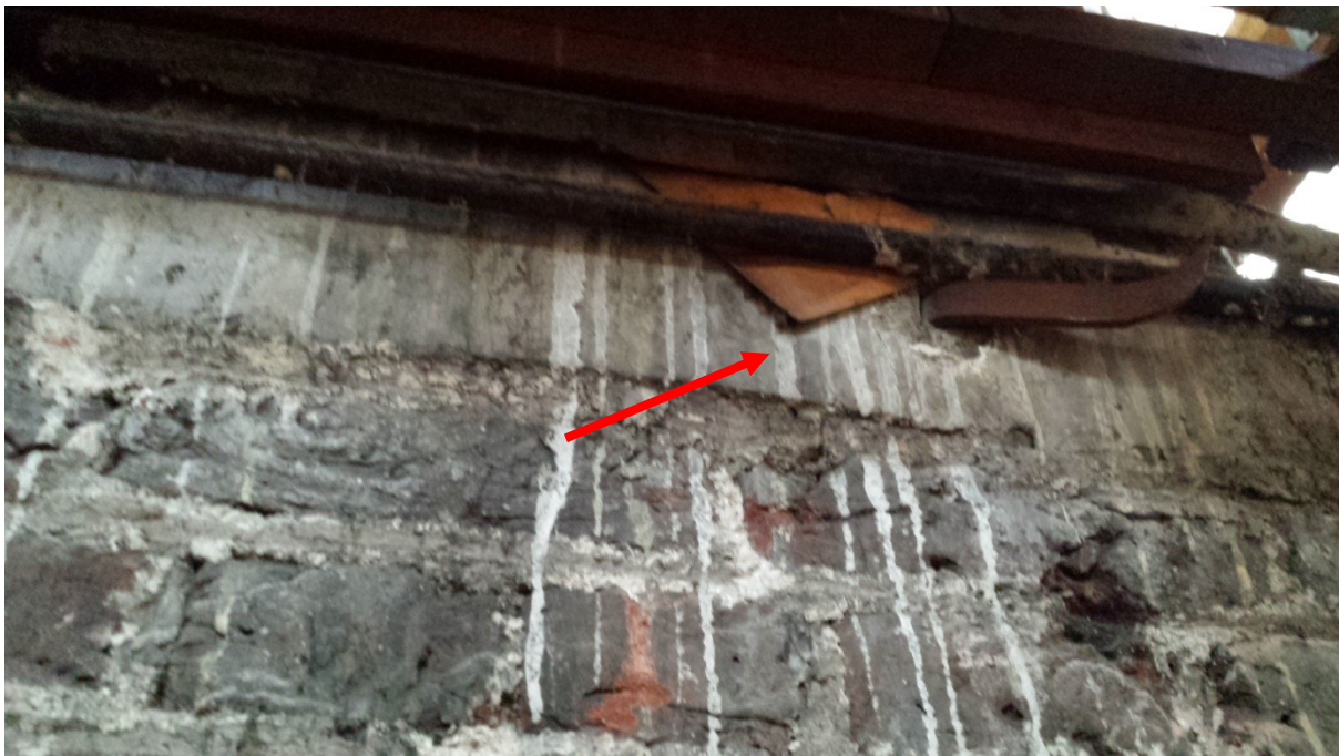
Figure 39 North wall - Bookcase 17 - traces of plaster and paint
