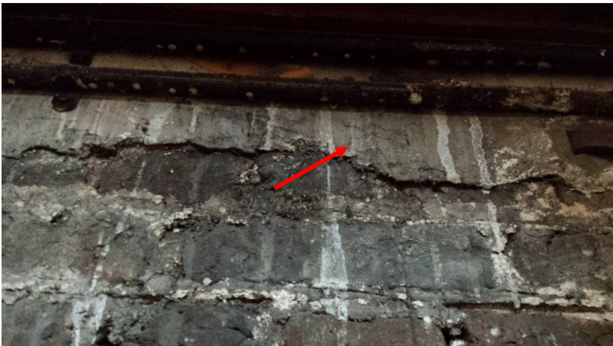
Figure 38 North wall - Bookcase 13 - traces of early plaster and paint
