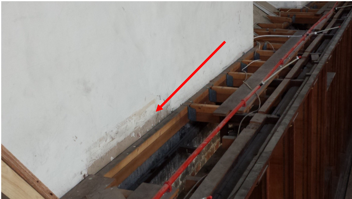
Figure 37 Geat Hall - Detail sof wall plaster
